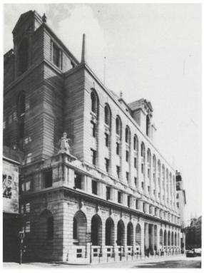
The main facade of Midland's head office at Poultry, London. The building was steel-framed with Portland stone elevations. The Poultry section was completed in 1930.
